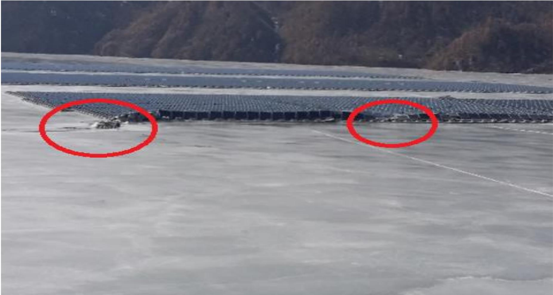
Ochang Reservoir Solar module damaged caused by ice pressure
