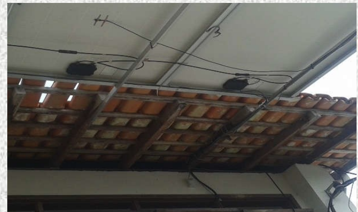
Air and module temperature sensors
