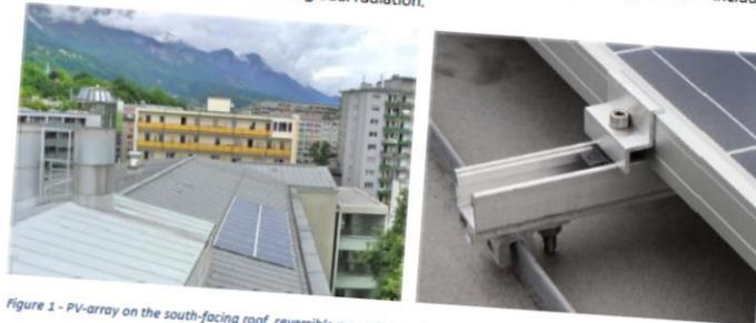
Figure 1 - PV-array on the south-facing roof, reversible mounting by the tin roof fold-clamps
